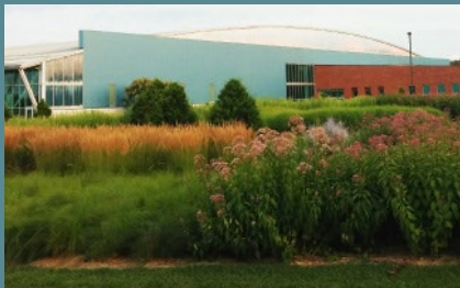
The Renaud Spirit Center received mechanical and electrical upgrades in Phase II, decreasing energy costs and providing reliable, long term systems.
