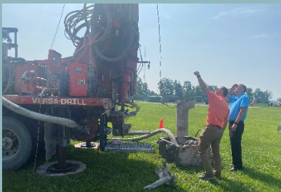
Geothermal Test Well Drilling
