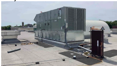
Ph. 2: The new, energy-efficient HVAC rooftop unit installed atop the Julia Davis Location
