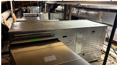
Ph. 3: Installed new energy-efficient Geothermal HVAC system at the Carpenter location (above & below).
